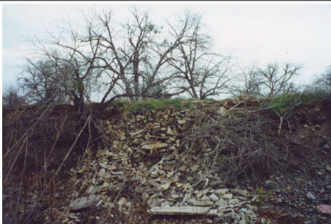
Photo 3.5: Example of informal bank protection measures.
