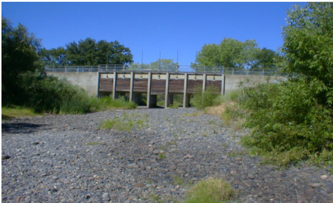
Photo 1.3: Lindo Channel Dam at the Head of Sandy Gulch
