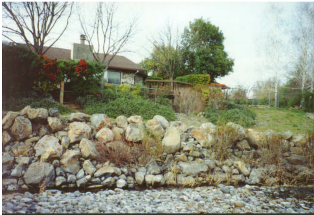
Photo 3.3: Rip-rap in place as bank protection measure.
