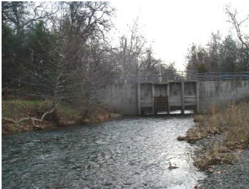
Photo 1.1: Box culverts regulating flow on Big Chico Creek into Sandy Gulch.
