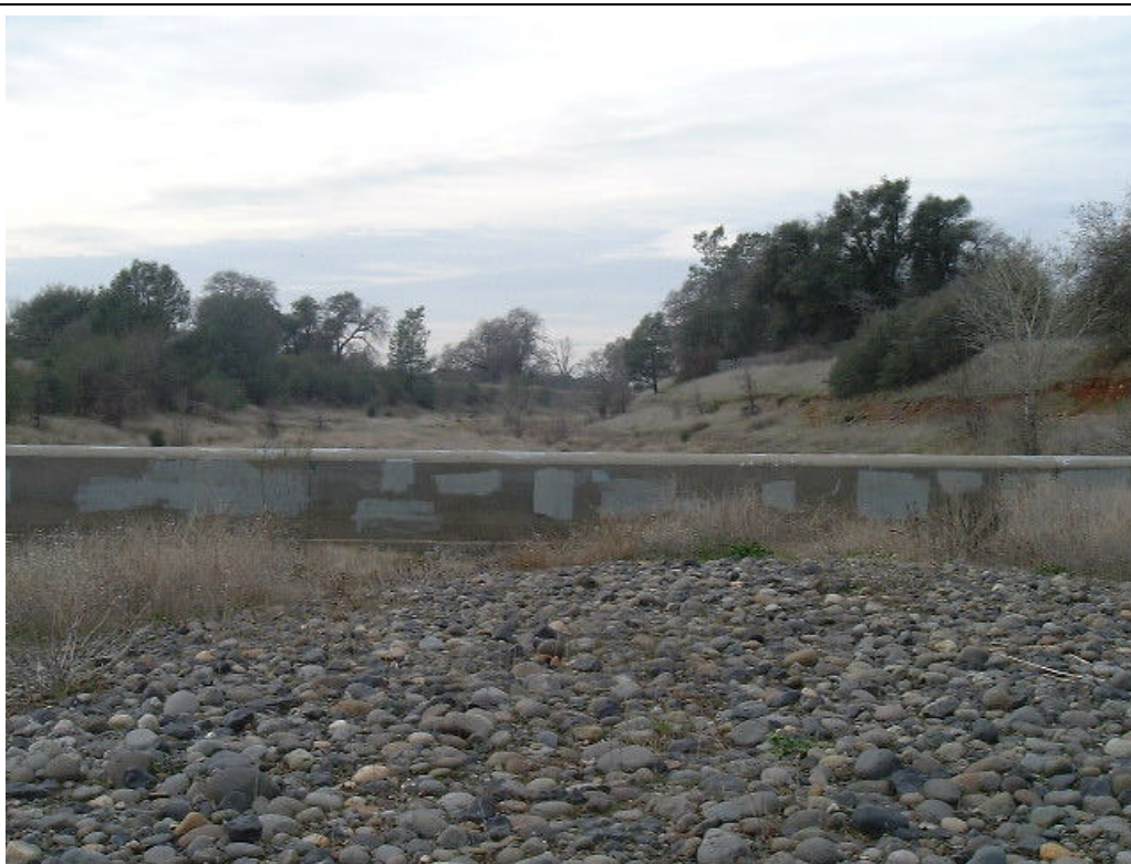
Photo 1.2: Concrete weir controlling flow into the Sycamore Creek Diversion Channel
